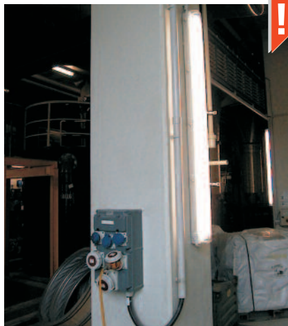
Vertical wall mounting with lampholder supports
