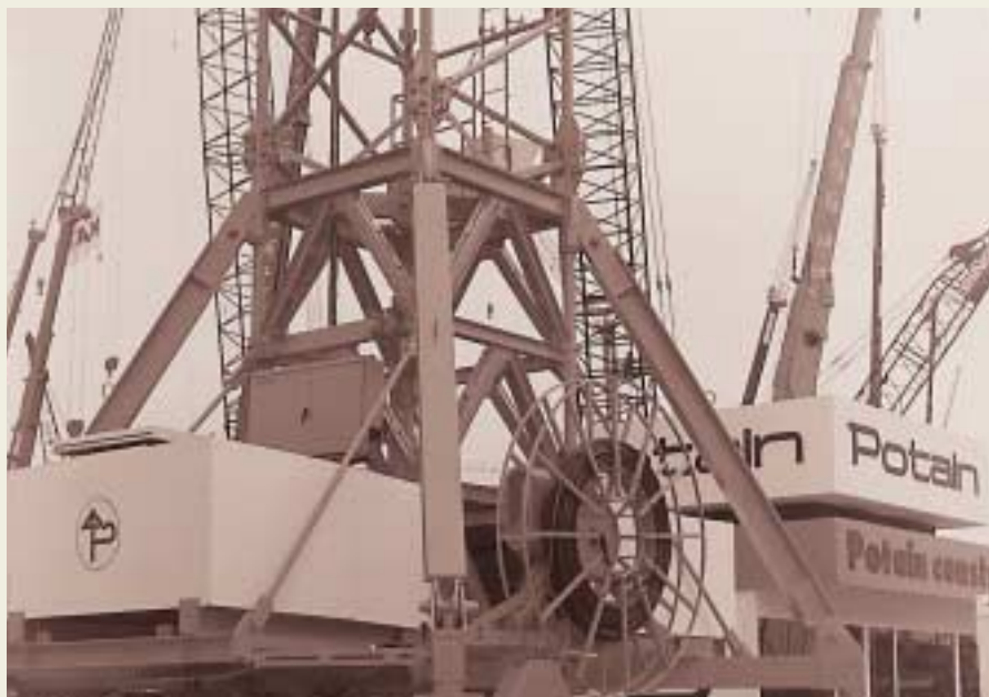
Potain tower crane - 1966.
