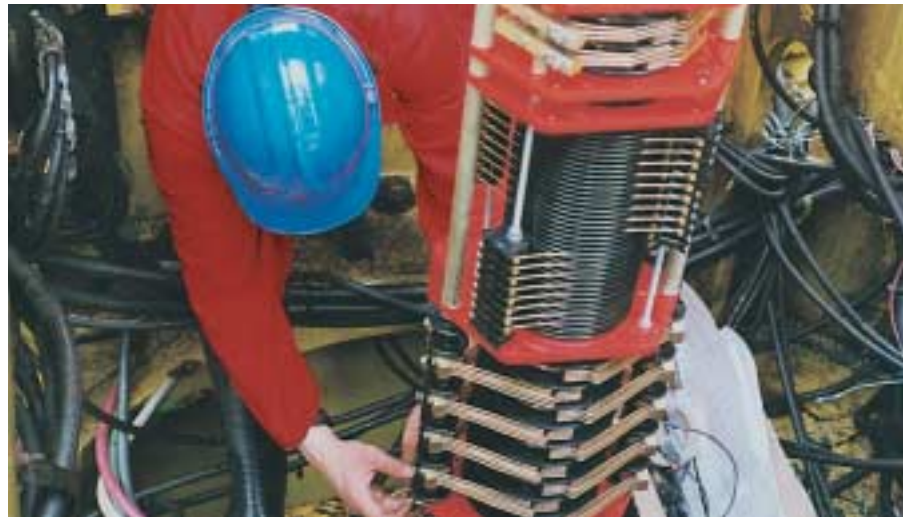
Replacement of a damaged slipping unit on an offshore application in Qatar, at +48 deg. C
