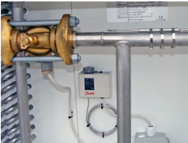
1'000 kg/h (2'204.62 lb/h) atmospheric ASCO CO 2 Vaporiser: Thermostat
